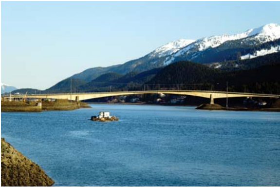
Juneau Douglas post-tensioned bridge over the Gastineau Channel in Juneau, Alaska. (Photo courtesy of SCS)
