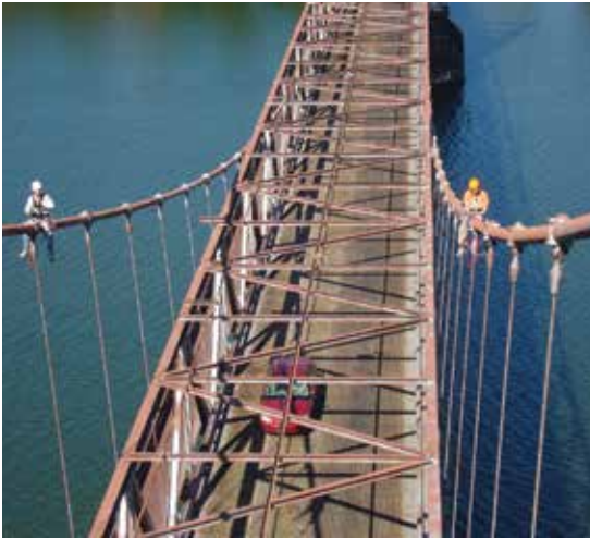
Above: Specially trained Burgess & Niple engineers used rope access to inspect the towers, cables, and trusses without closing the bridge to traffic. Right: The 1,704-foot-long Market Street Bridge, shown here before rehabilitation, was constructed in 1904 and had undergone several modifications during its life but had not had many repairs since the 1980s.
