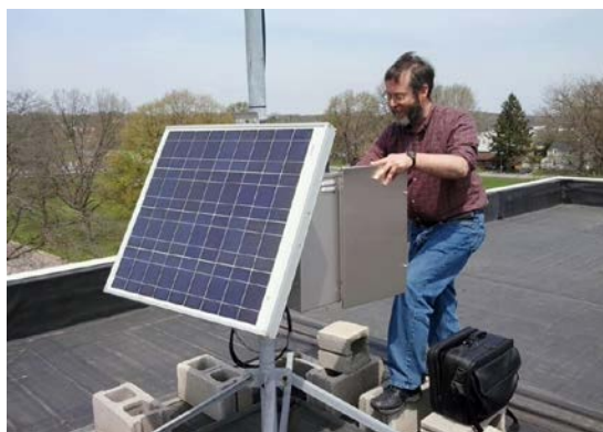
40 DCUs receive radio signals from 40,000 MTUs and send data via cell phone to Utility Billing System Database
