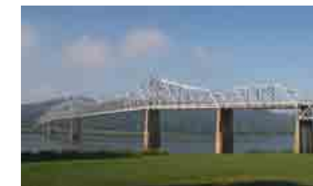
Pictured Above: The existing Milton-Madison Bridge.
