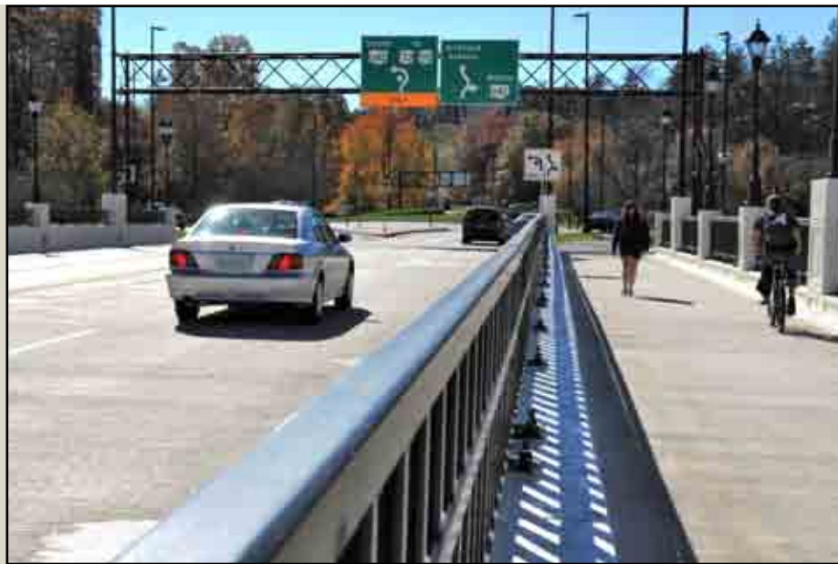
The barrier-separated pedestrian and bike pathway on the Richland Avenue Bridge in Athens, Ohio provides separation from vehicles and a safer bridge crossing. Enhanced safety for all travelers was the intent of the major structural and aesthetic improvements made to the bridge.
