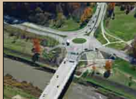
Pictured Below: An aerial view of the Richland Avenue Corridor Improvement Project.
