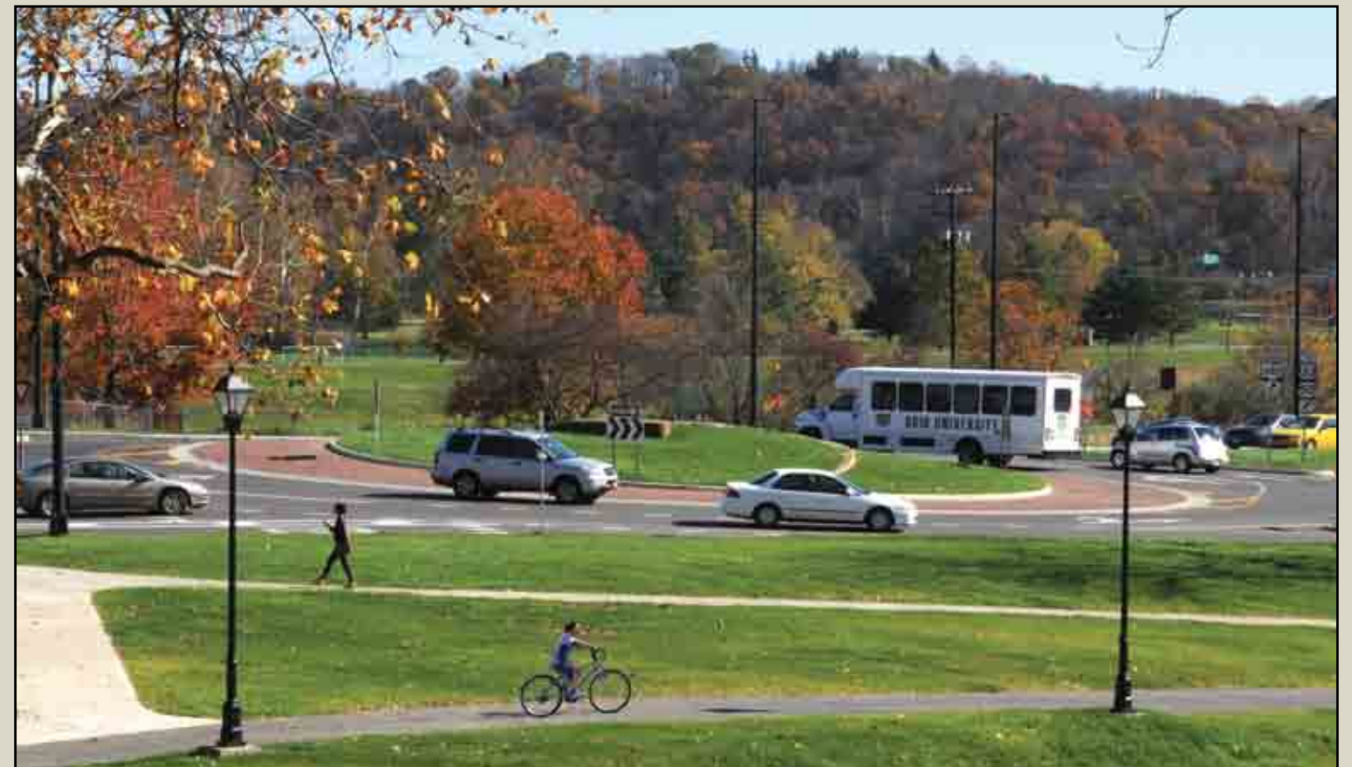
Multimodal mobility and safety is at the center of a newly designed corridor in Athens, Ohio. Pedestrians and bicyclists travel on dedicated, ADA-compliant pathways while the new multilane roundabout is large enough to easily accommodate vehicles including buses and tractor-trailers.
