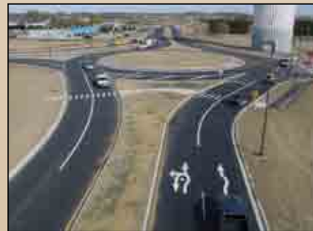
Pictured Above: The new SR 161-Post Road/Industrial Parkway roundabout.
