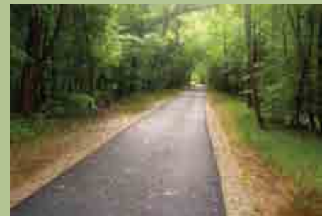
Pictured Below: B&N provided civil engineering services for this Fairfax County trail.
