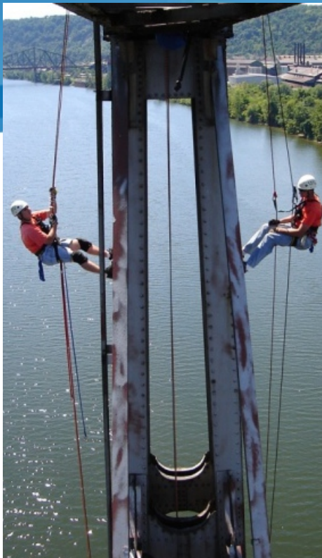
Figure 6 – Tower Inspection by Rappelling
