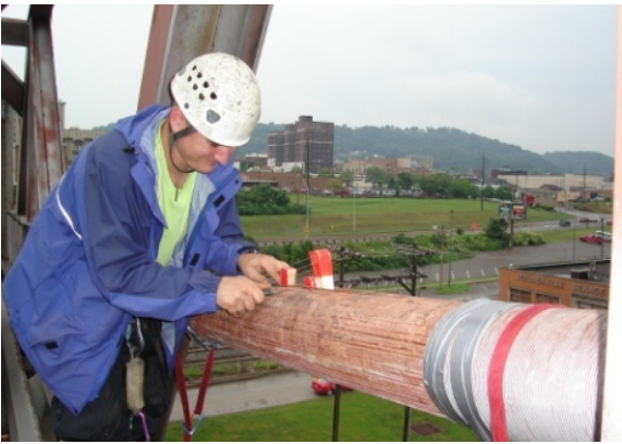
Figure 9 – Strand Inspection
