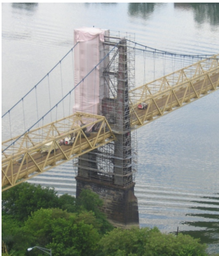
Figure 17 – Tower Containment
