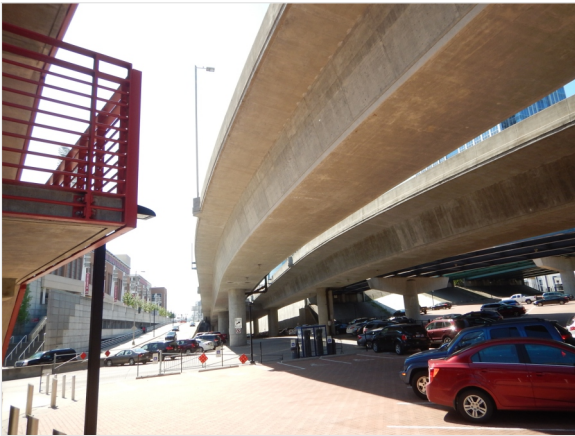
This ramp from Second Street to EB US50 over Broadway in Cincinnati, OH, is a five-span structure with internal PTS in the webs and CIP.
