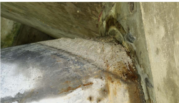
Soft grout can be seen at the anchor of the steel tendon pictured here. (Photo courtesy of VSL)
