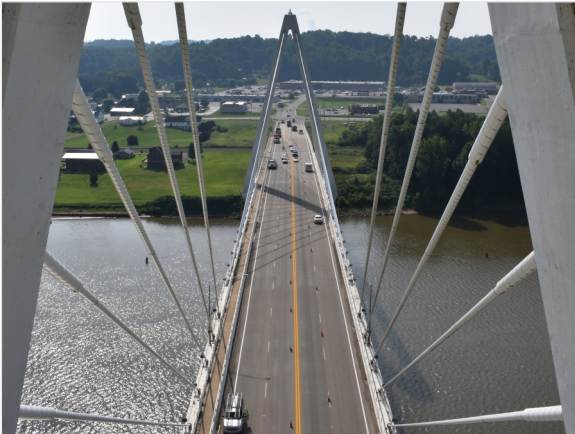
Bridge of Honor Cable Stay Bridge over the Ohio River between Mason County, West Virginia and Meigs County, Ohio.
