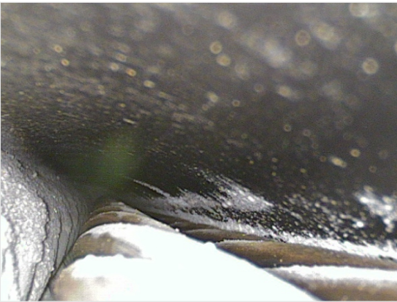
External PTS duct: An incomplete grouting procedure has resulted in voids and corrosion of the exposed strands.
