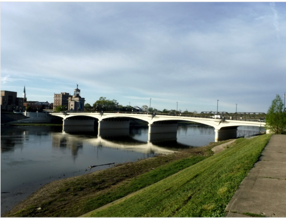
The State Route 129 bridge over the Great Miami River in Butler County, OH includes internal PTS, precast haunched girders.
