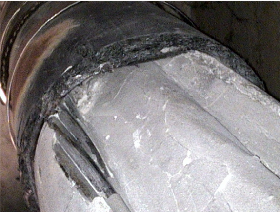
External PTS duct: Note that the steel tendon is partially exposed and has voids indicating an incomplete grouting procedure.
