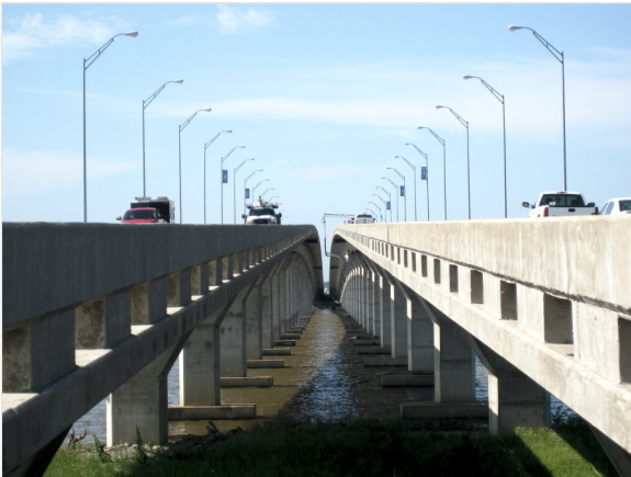
The twin Sailboat Bridges carry US 59 over Grand Lake in Delaware County, Oklahoma. Twenty-five spans comprise each structure and are supported by external PTS.
