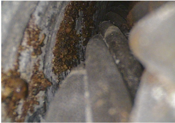
This tendon duct has no grout. Note that there is rust on the duct interior and the steel tendon strands. (Photo courtesy of VSL)
