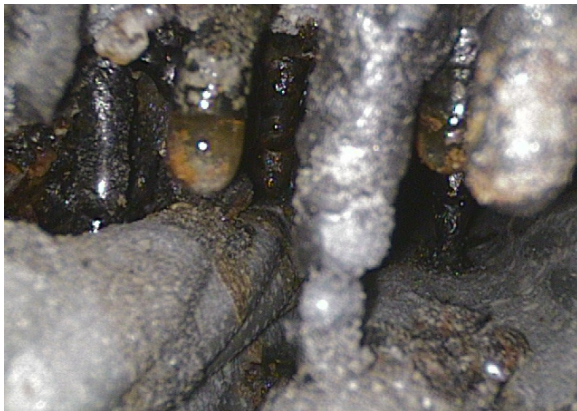
This image shows a duct with exposed tendons in the duct interior. Note the mineral and water deposits. (Photo courtesy of VSL)
