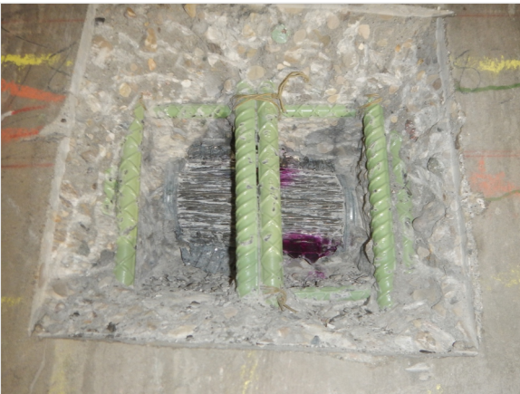
This exposed internal steel tendon has a 1" void at the top of the duct. The purple colored areas have been sprayed to confirm that the pH of the grout is 12 to 13.
