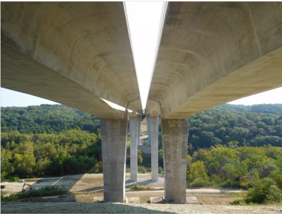
The twin Jeremiah Morrow bridges carry I-71 over the Little Miami River in Warren County, OH. Internal and external PTS, CIP segmental box construction.
