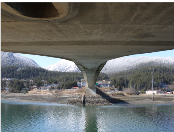
The Juneau Douglas Bridge Road over the Gastineau Channel in Juneau, Alaska, consists of an internal PTS box girder.
