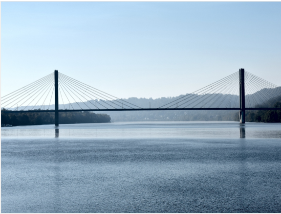
William H. Harsha Cable Stay Bridge over the Ohio River in Mason County, Kentucky.
