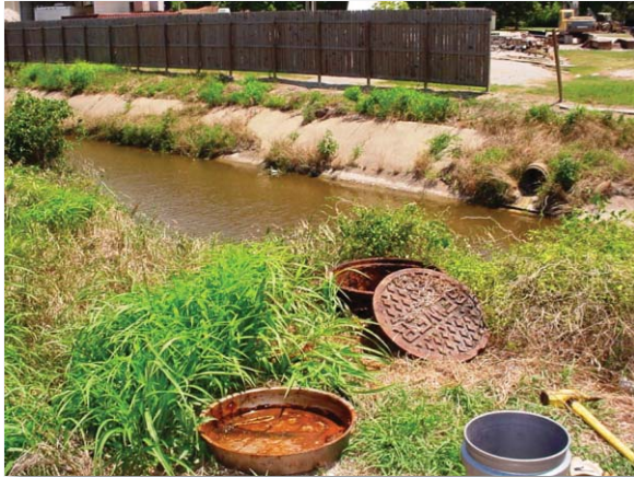
Figure 16.0 – Picture of Pipe in a drainage channel
