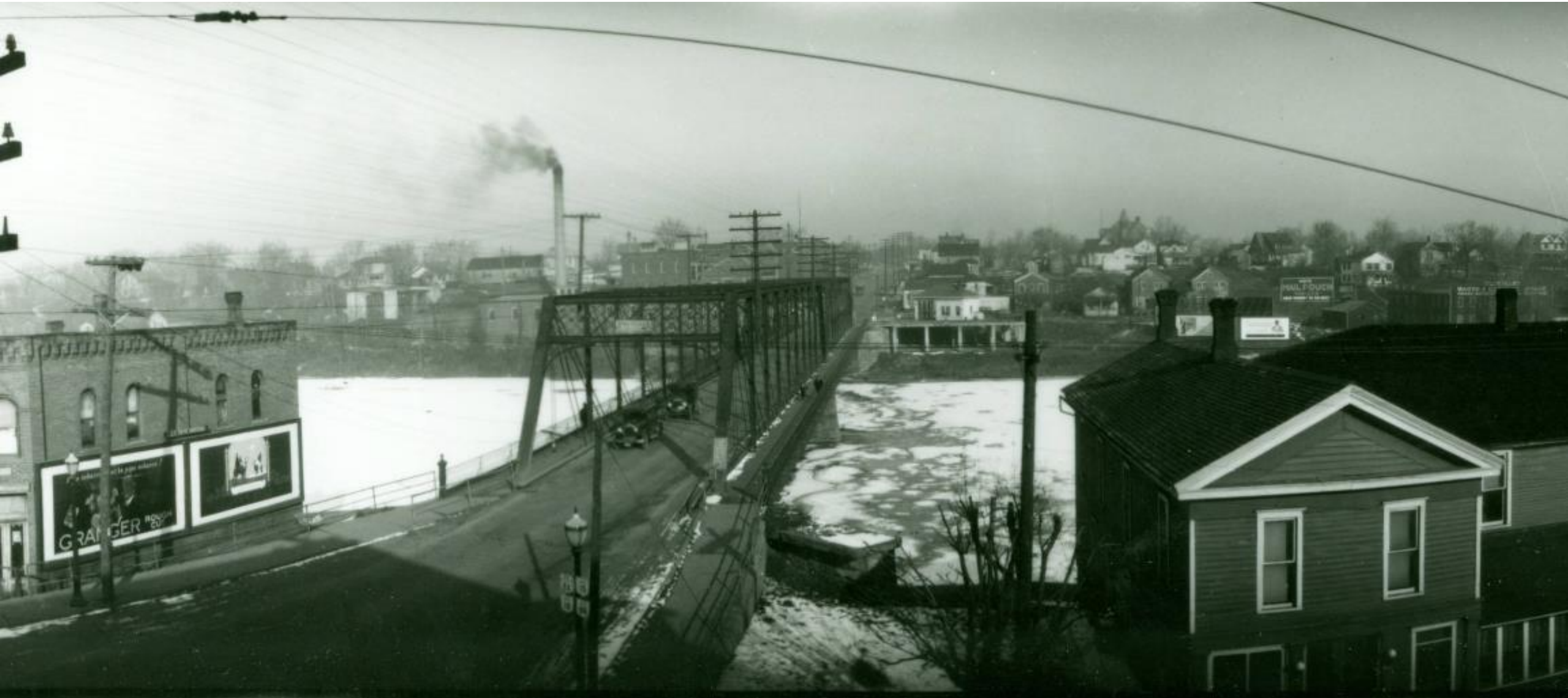
Two-Span Truss Bridge at Clinton Street, 1931
