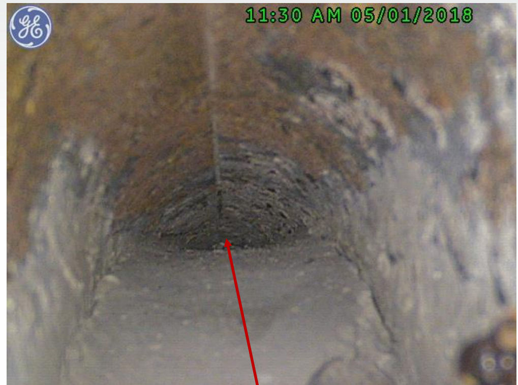
1/8 inch void between trumpet and grout vent
