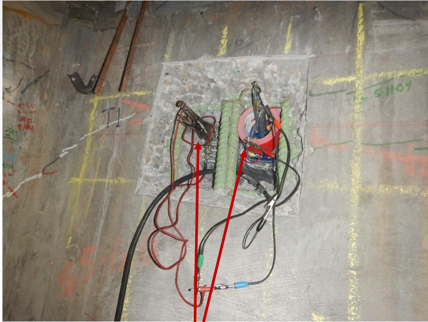
Typical corrosion rate set up, connecting directly to the tendon bundle
