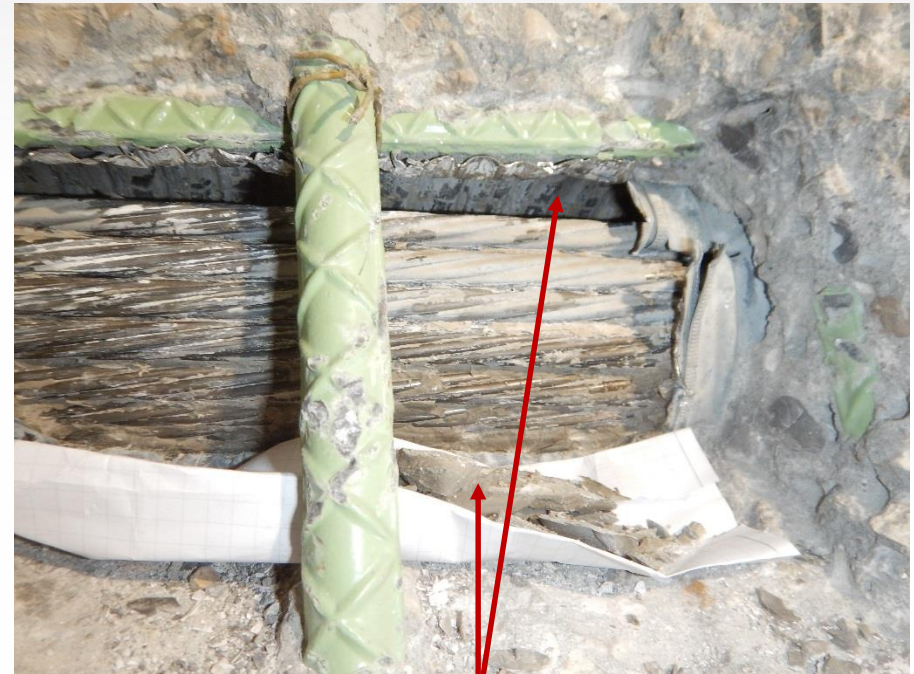
Typical grout sampling from the exposed tendon duct. Note void at top of duct
