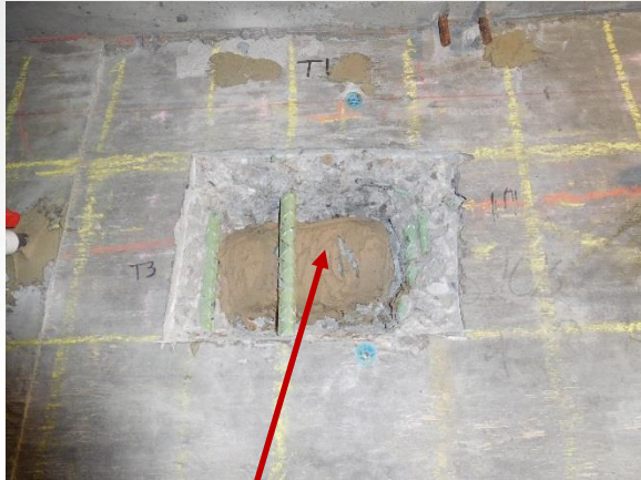
Repair of corrosion rate test location. Duct has been epoxied back into original location
