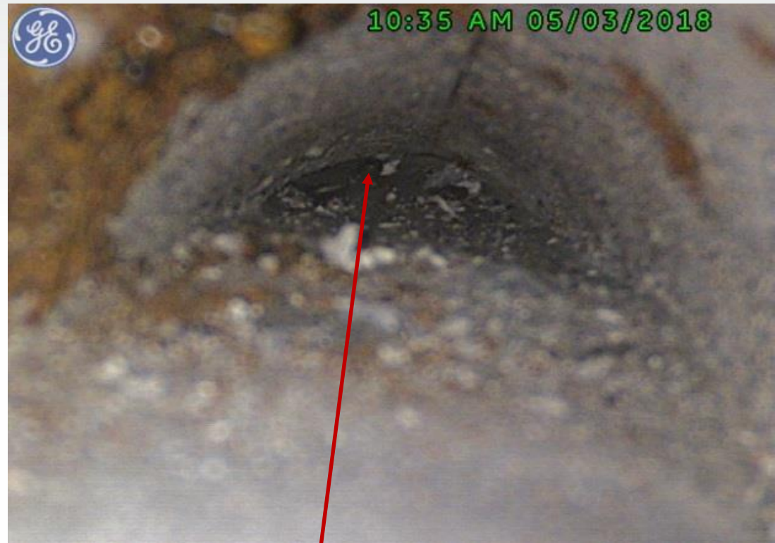
1/4 inch void between trumpet and grout vent
