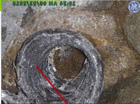
Entrance to empty grout vent and corrosion at vent interior
