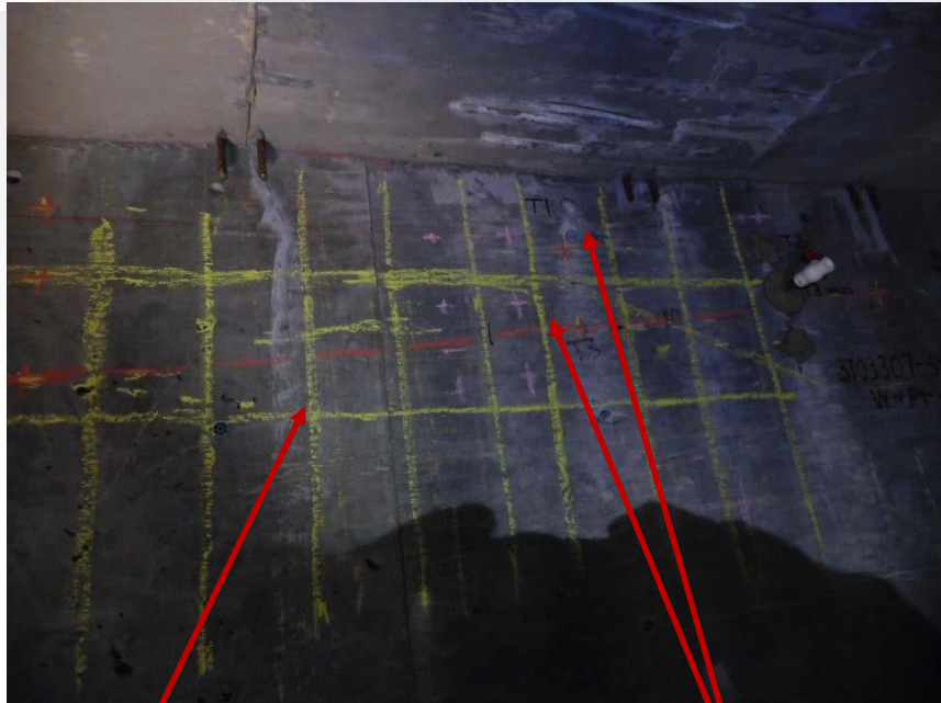
GPR located reinforcement steel
