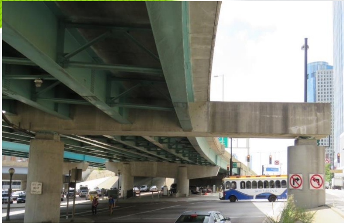
HAM-71-0111L over 3 rd St & Broadway PTS Pier Cap 2
