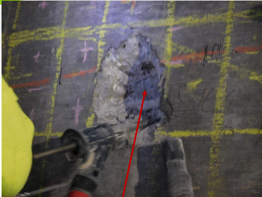
Chipping concrete to access tendon duct in web wall
