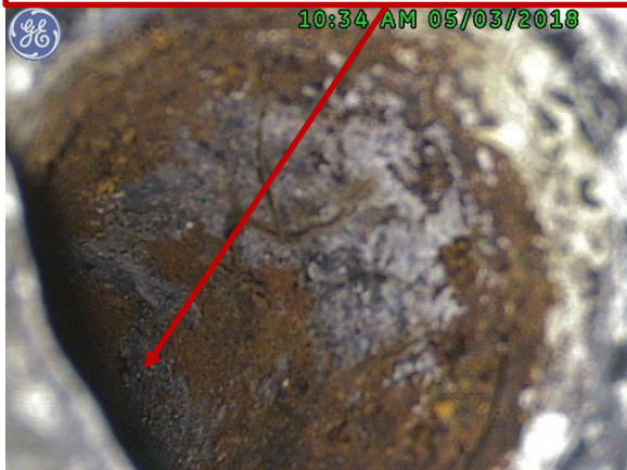
Entrance to empty grout vent and corrosion at vent interior
