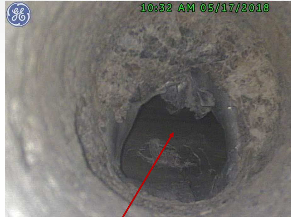
Looking into borescope test location, void at top of duct
