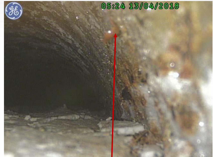
Void at highpoint with moisture corroding the duct interior
