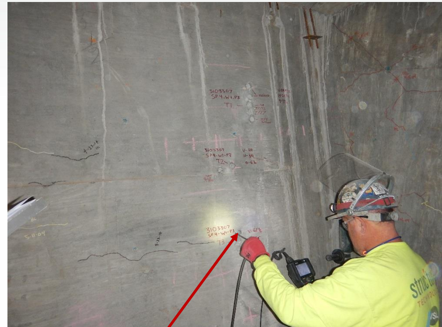
Inserting borescope camera line into test location
