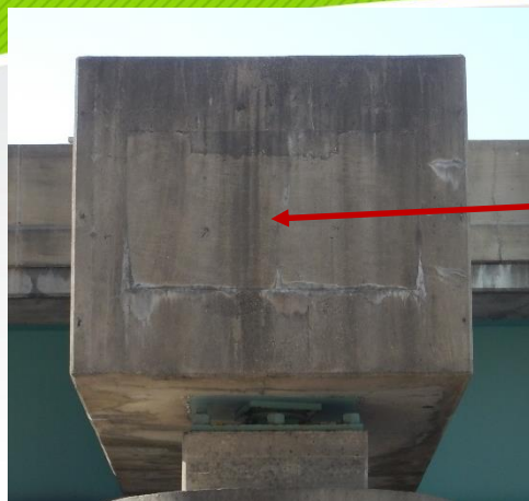
Blockout at north end of pier cap
