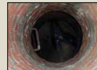
B&N's on site visits provide an up-close view and invaluable insight into existing conditions.
