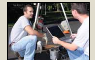
Flow meters and rain gauges supply important data used to pinpoint problem areas.
